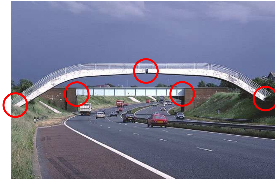
foto: Godden Structural Engineering Slide Library Courtesy National Information Service for Earthquake Engineering, University of California, Berkeley
