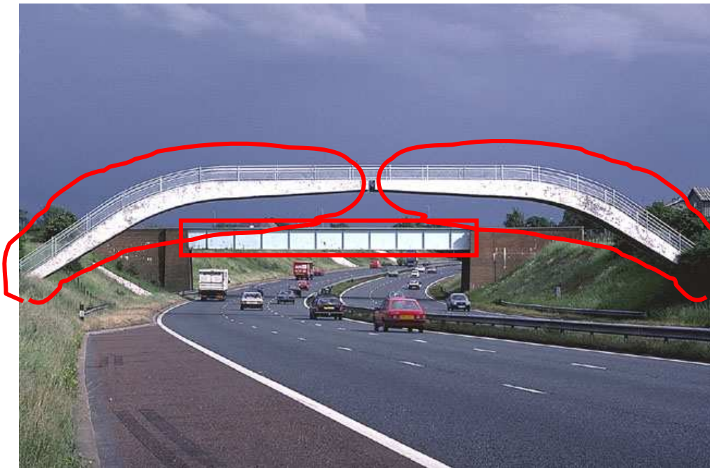
foto: Godden Structural Engineering Slide Library Courtesy National Information Service for Earthquake Engineering, University of California, Berkeley
